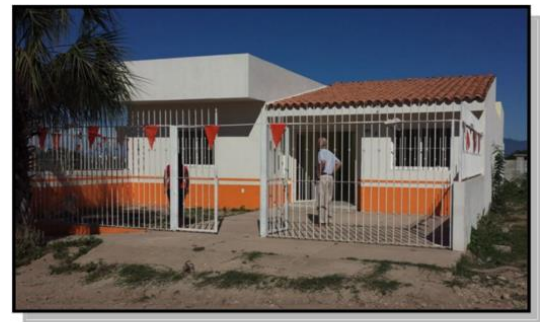
Existing Sewing Sewing School Building
